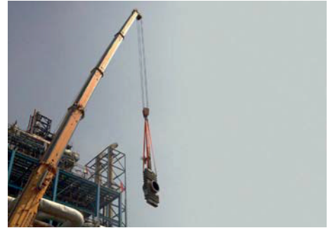
Valve being hoisted into position
